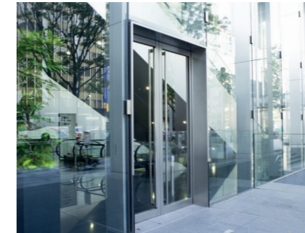
IP & ENTRANCE PANEL CAMERA MONITORING
