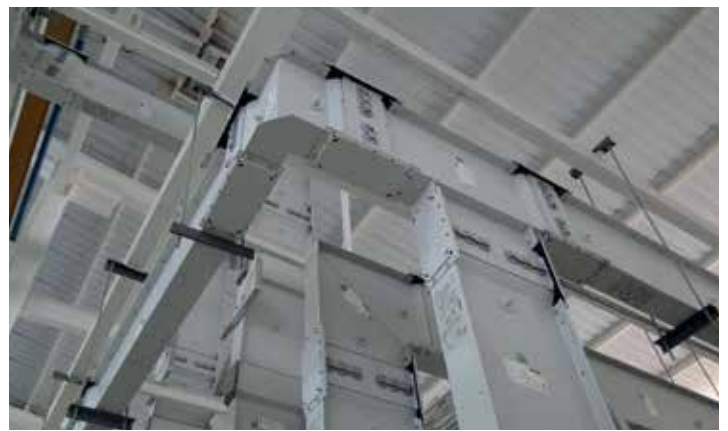
Example of Legrand busbar system
