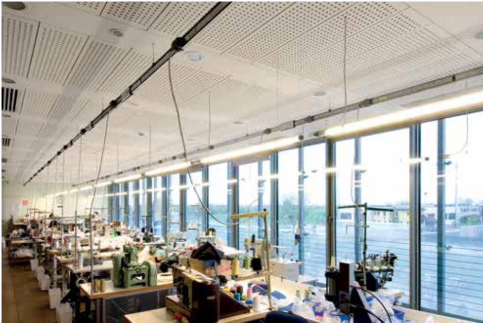
Example of lighting and small power distribution
